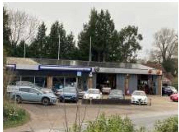
The new solar array
