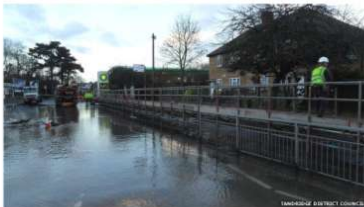
A scaffolding bridge has been built over the flood water to give residents a walkway
