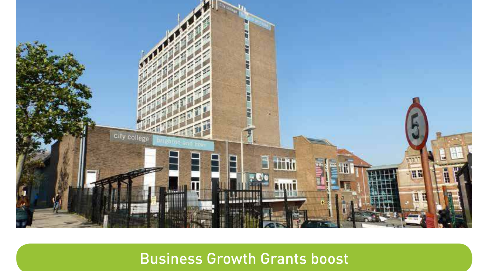
Affordable housing in Redhill
